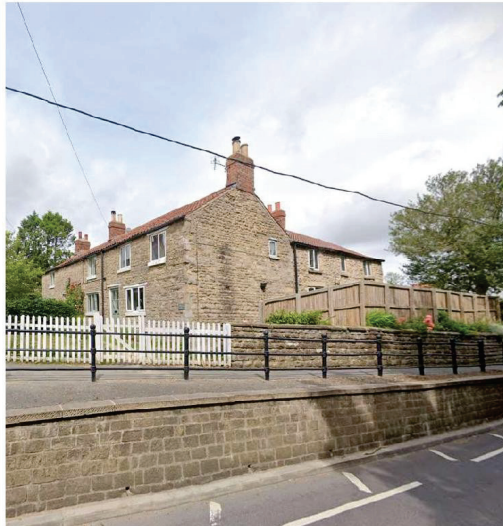
Example of a retaining walls along Amotherby Lane, which is in close proximity of the proposed site
